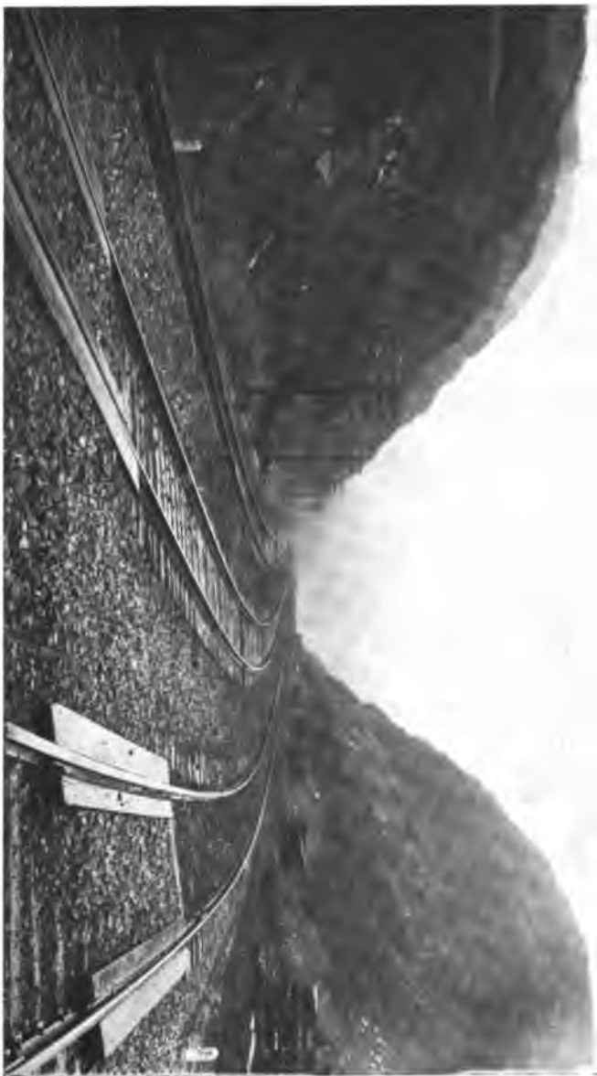
View of the three-track line of the Baltimore and Ohio Railroad in Preston County, showing the open cut which has taken the place of McGulpre's tunnel.
